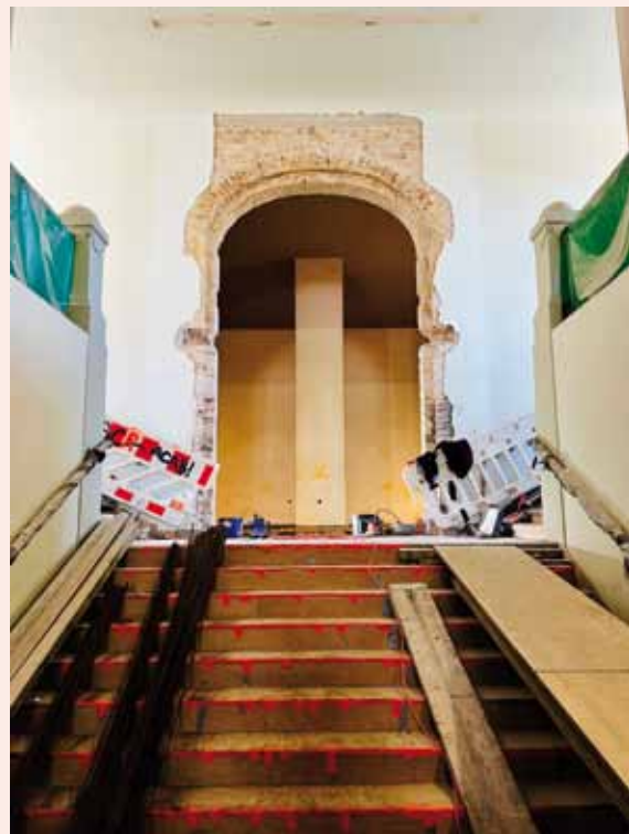
View through the almost five-metre-high archway into the Engler Hall.
